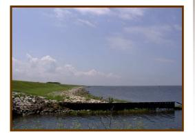
The Herbert Hoover Dike System (HHD) consists of approximately 143 miles of earthen embankment located along the perimeter of Lake Okeechobee.
